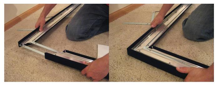
Confirm with your fingers at the joint that they are perfectly joined and then start tightening the set screws. Please use the ball-point end of the wrench we provided so that you can more easily access the screws and won't over tighten them. Their cup points will bite into the aluminum, securely locking the frame to the steel corner brackets.
