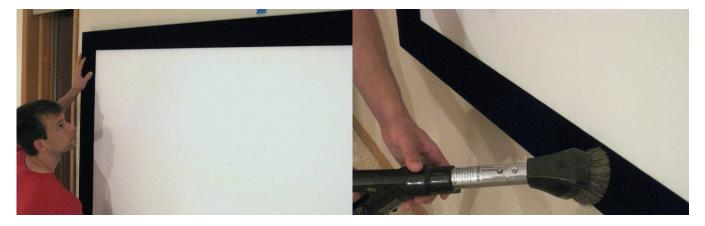
The installation shown clearly has surfaces that are lighter than a medium shade. Because the Center Stage XD screen has 1500 tiny holes per square inch, you'll need all the surfaces behind the screen to be a medium color or darker, and reasonably non-reflective. If you can't paint everything dark, then you can easily add a secondary black backing layer. It installs just like the screen, just with fewer grommets and o-rings since that layer doesn't need much tension.
